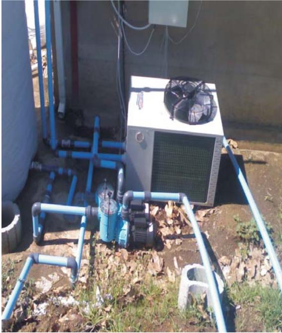
*Figure 2 Heat pump and storage tank*
